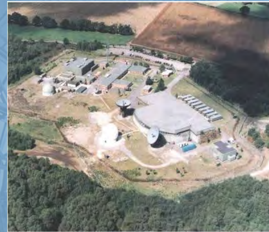
Oakhanger Satellite Ground Station
